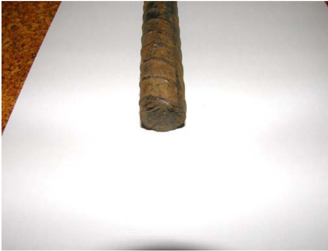
Figure 1a. Rebar SCC.
