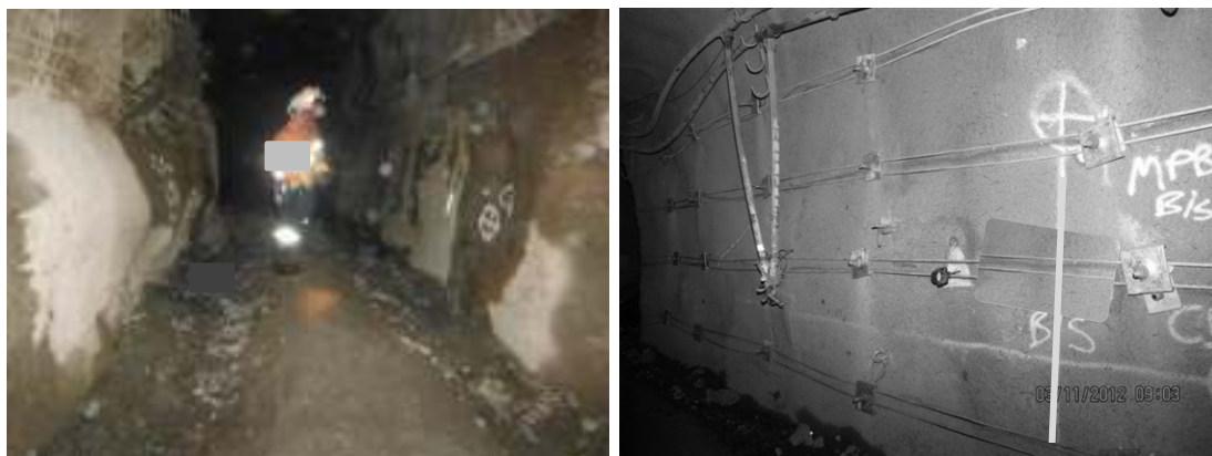
Figure 16 JTech Bolt and surface support for squeezing ground
