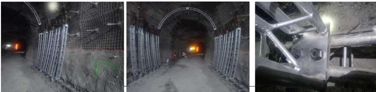
Figure 16 Installation of legs for the Lattice Girders
