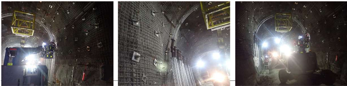
Figure 17 Installation of top arch members for the Lattice Girders
