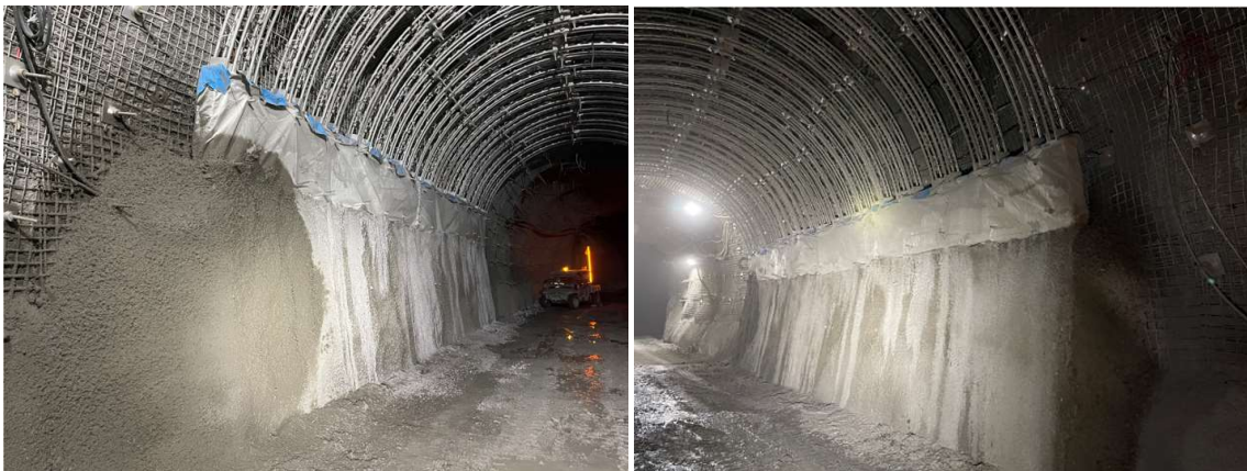
Figure 19 The Lattice Girders are fully installed, yielding joints are covered, the Lattice Girders are ready to be embedded into fibercrete
