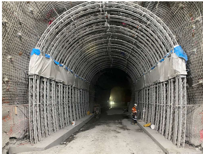
Figure 19 The Lattice Girders are fully installed, yielding joints are covered, the Lattice Girders are ready to be embedded into fibercrete
