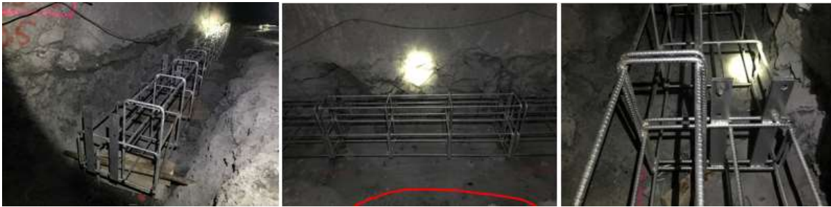
Figure 15 Construction of footings for the Lattice Girders
