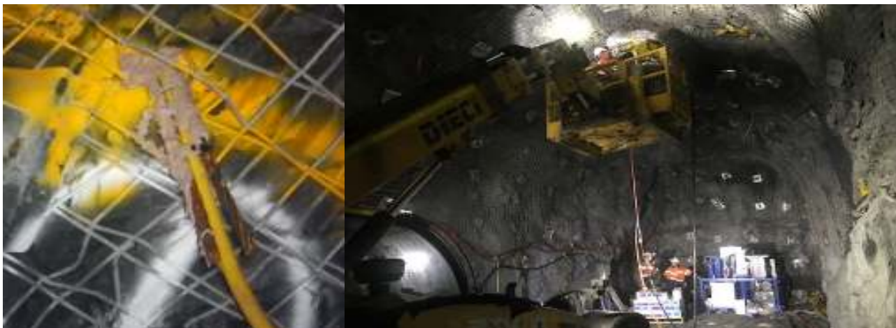
Figure 10 SECTA cable installed using traditional installation methods and J-Lok P resin
